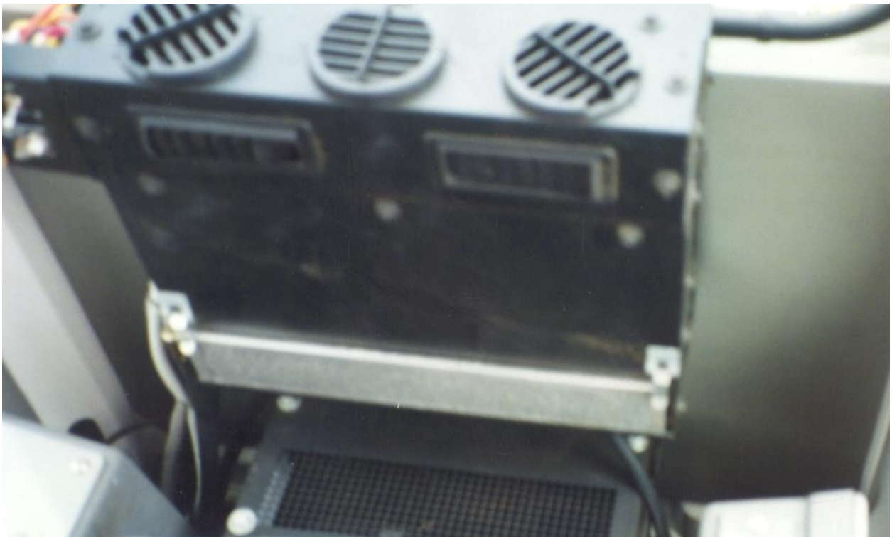
Evaporator assembly mounted in place.
